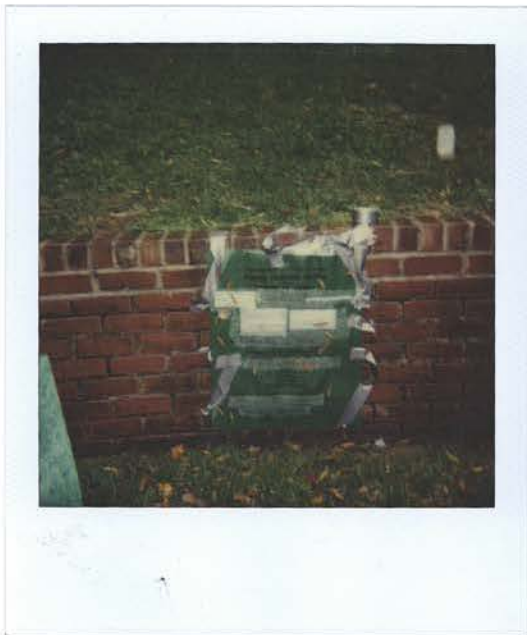
3. 11/12/02 – Replaced one sign - Western Ave., NW
